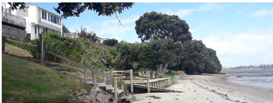
Figure 5-25: Knights accessway showing timber steps down to beach
