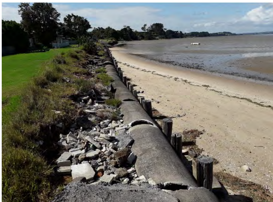
Figure 5-14: Glenbrook beach seawall and beach front
