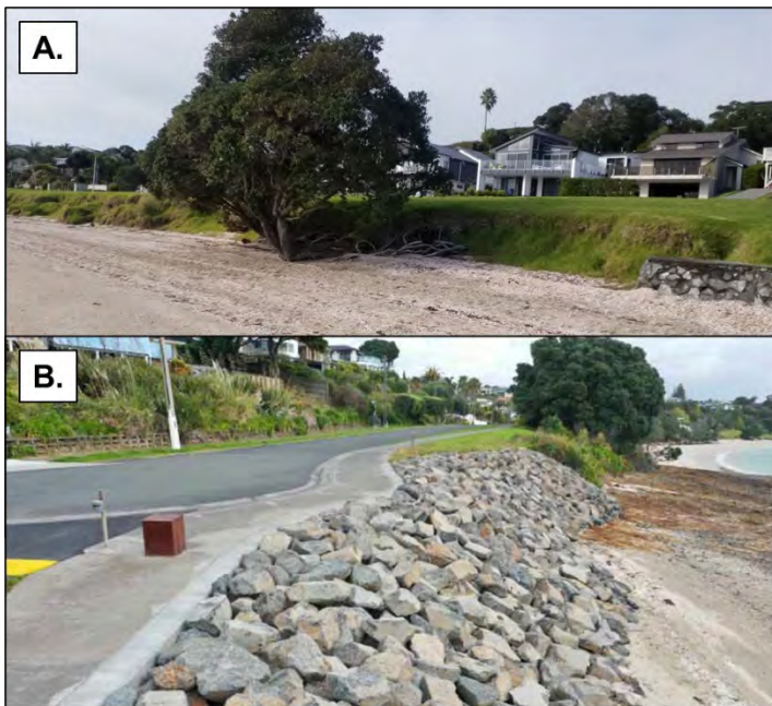
Figure 22: Photo of low-lying cliff edge (A) and the revetment protecting Te Pene Point (B)
