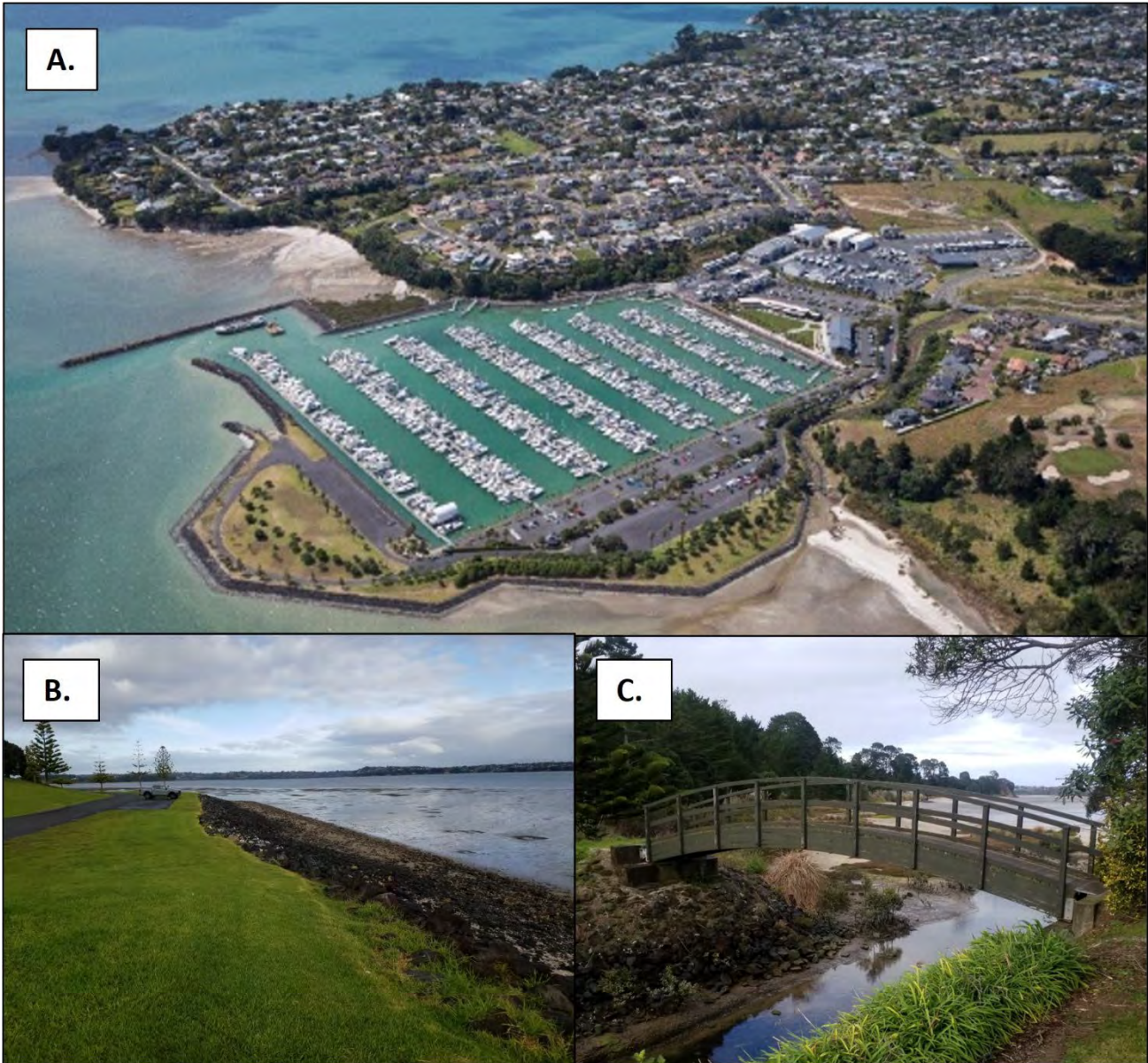
Figure 14 A) Aerial view of Kahawairahi/Pine Harbour marina, B) western revetment (photo facing south), C) pedestrian bridge linking the carpark to Kahawairahi/Pine Harbour Beach
