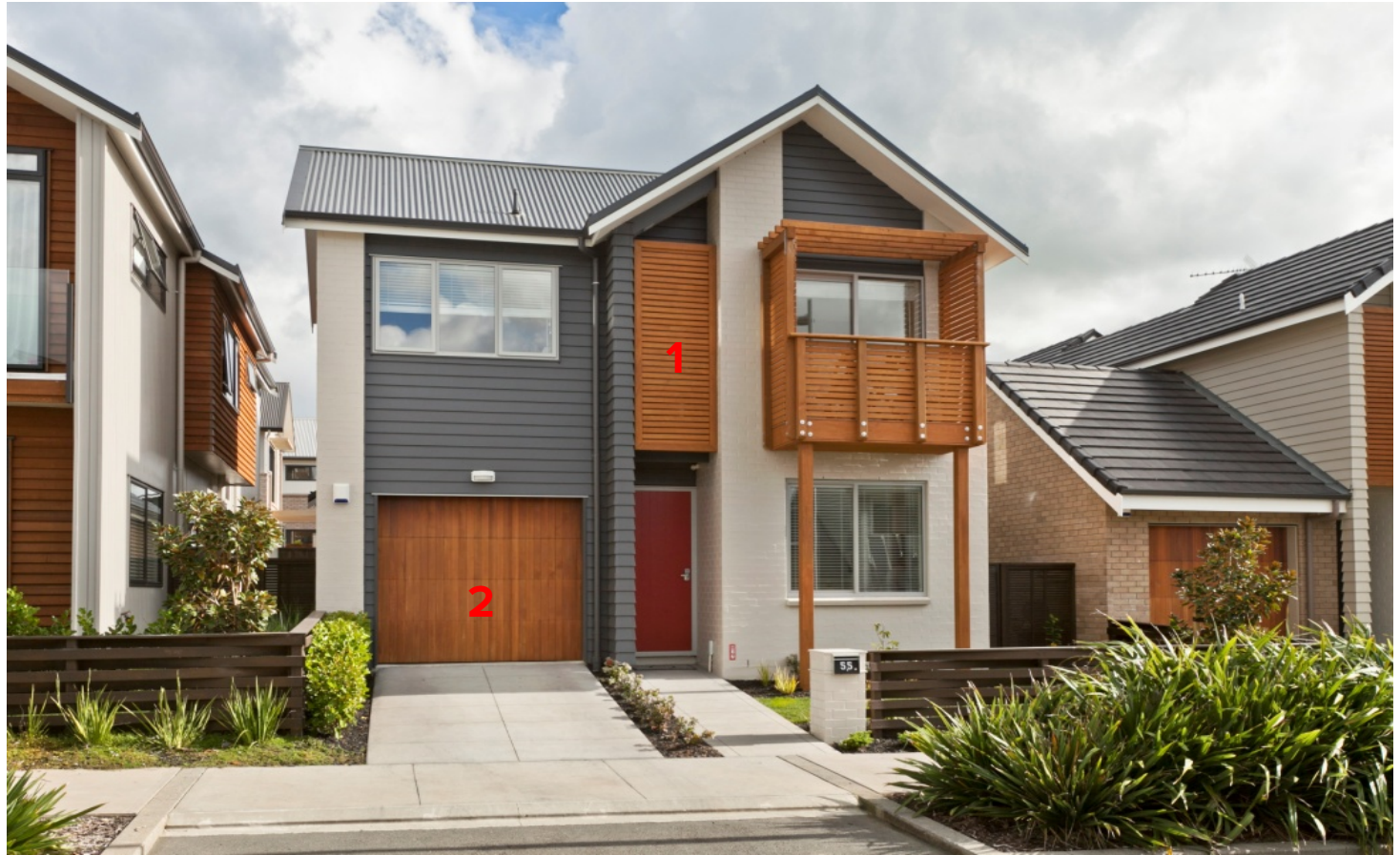
Looking towards the south elevation from Lester Street.
