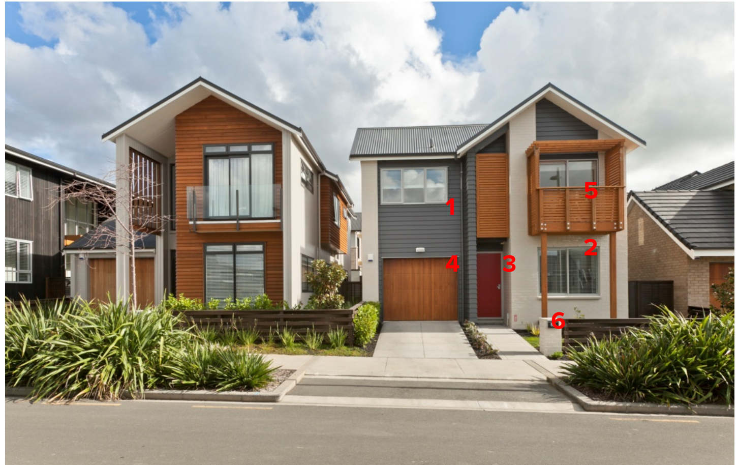
Looking towards the south elevation from Lester Street.
